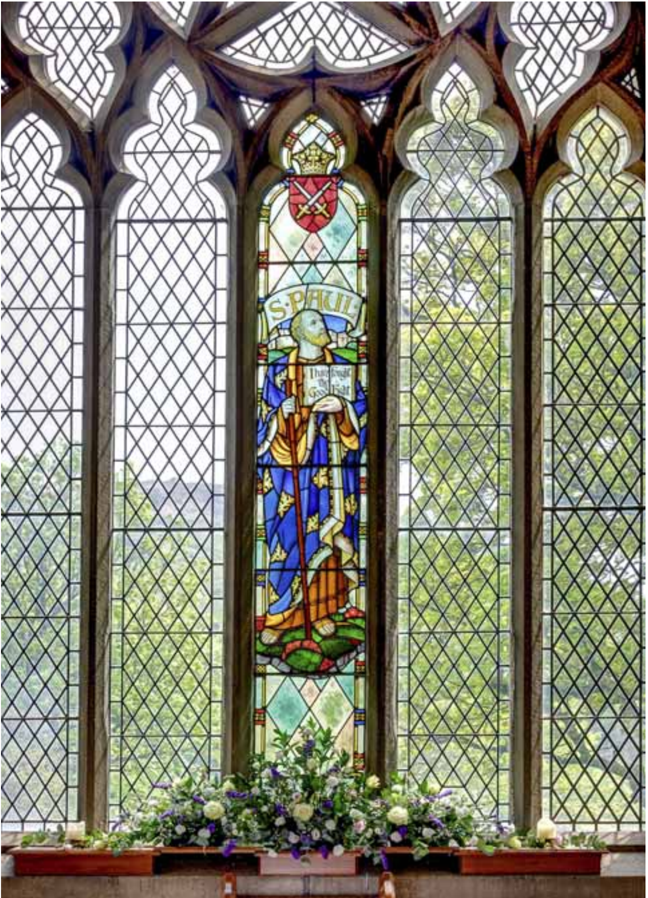
The stained glass window added to the South Transept in 1949.
