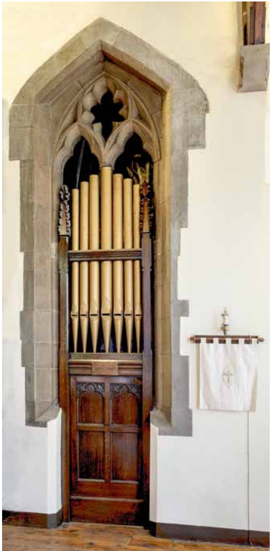
Door access to the organ pipes with 'dummy pipes' above.
